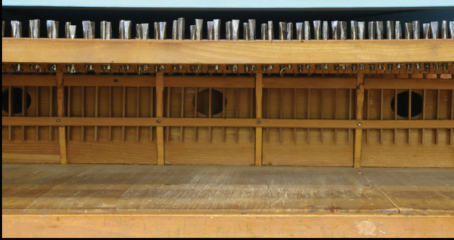
The inverted wrestplank, above: Cristofori piano 1726 underneath: G. Silbermann piano 1749
