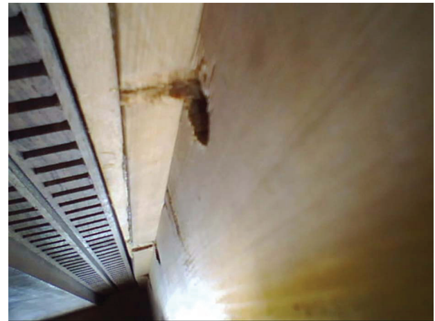
ill. 16, view underneath the registers, added strip to change the angle of the registers
